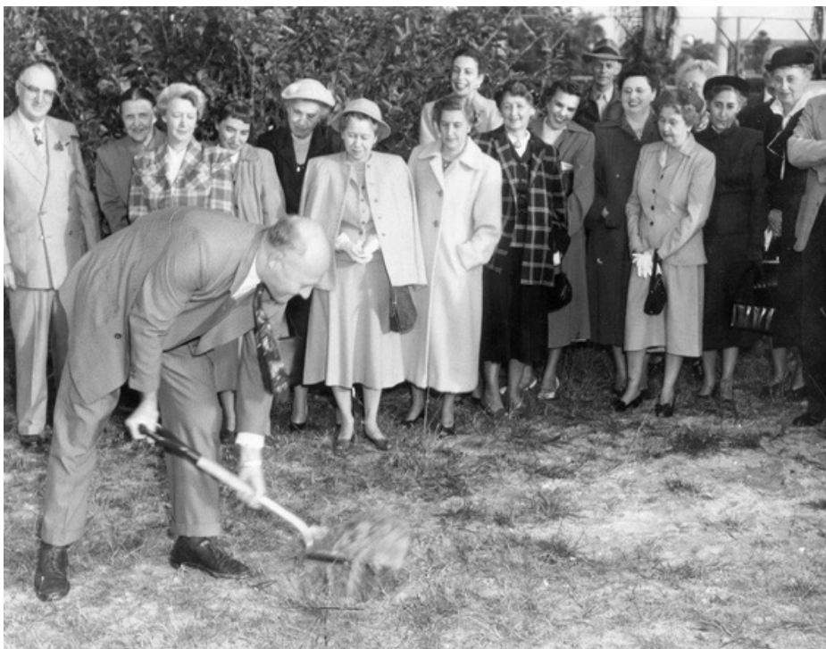
BWC Members at the ground breaking for the Manatee Players Club building
